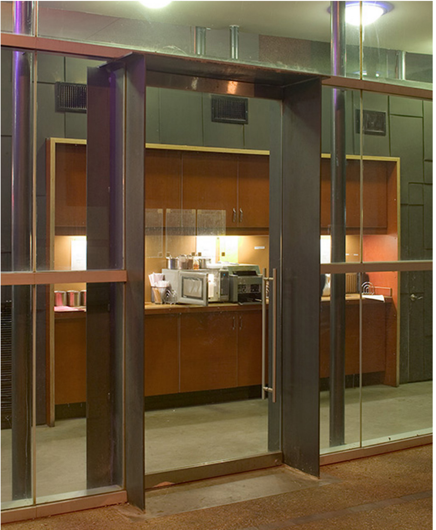
an extruded steel frame with pivot door marks one of the two entrances to the shop along the curving glass wall
